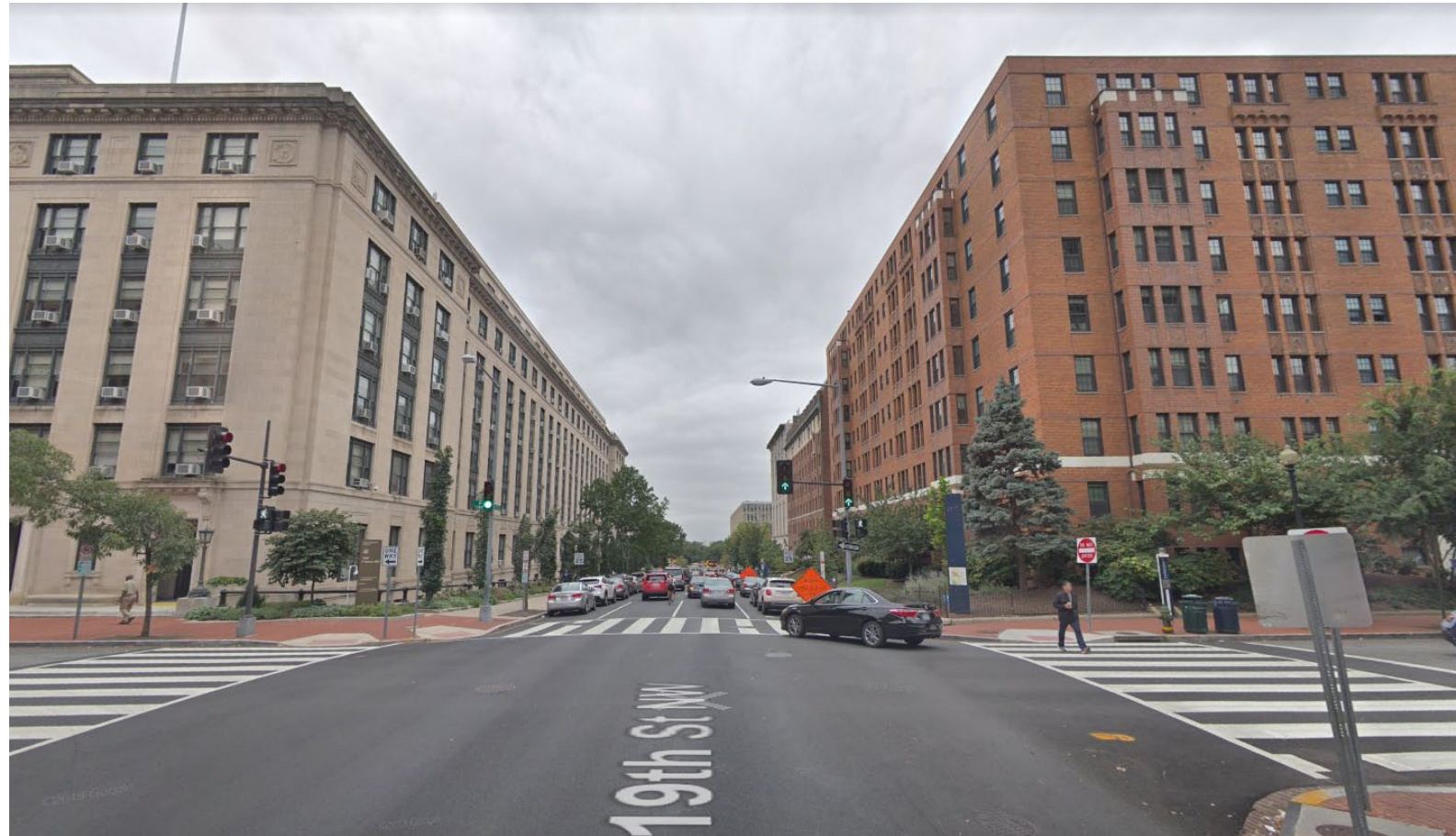
4. LOOKING SOUTH - 19TH STREET
