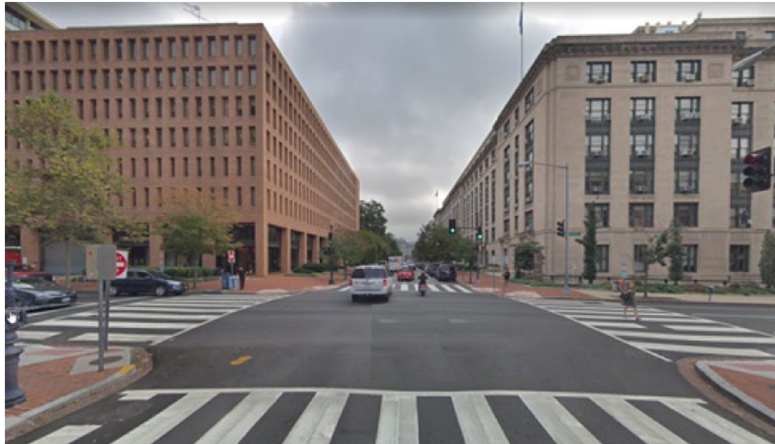
1. LOOKING EAST - F STREET
