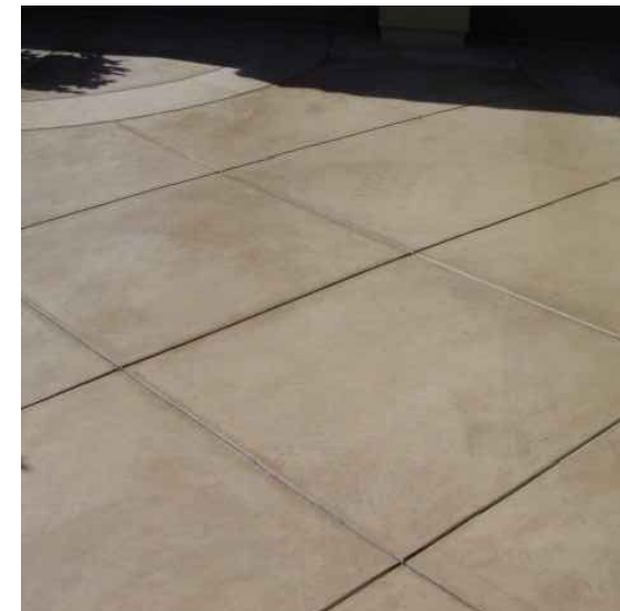
SCORED CONCRETE PAVING
