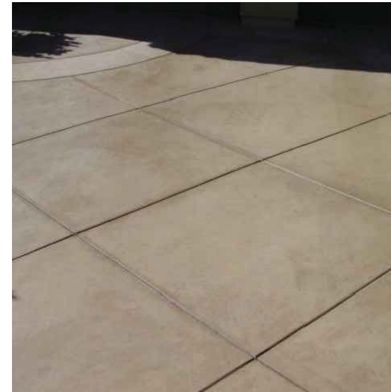
SCORED CONCRETE PAVING
