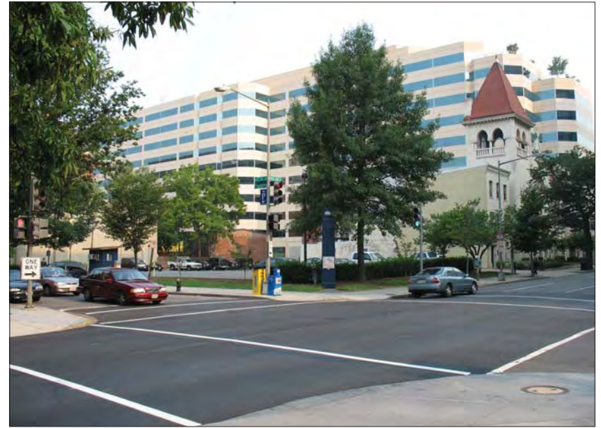
(3) Square 101: View north up 20th Street from H Street
