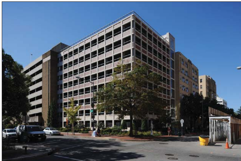
7.) Eye Street looking Southwest toward Parking Garage (demo.), with Munson and JBKO Residence Halls (right)
