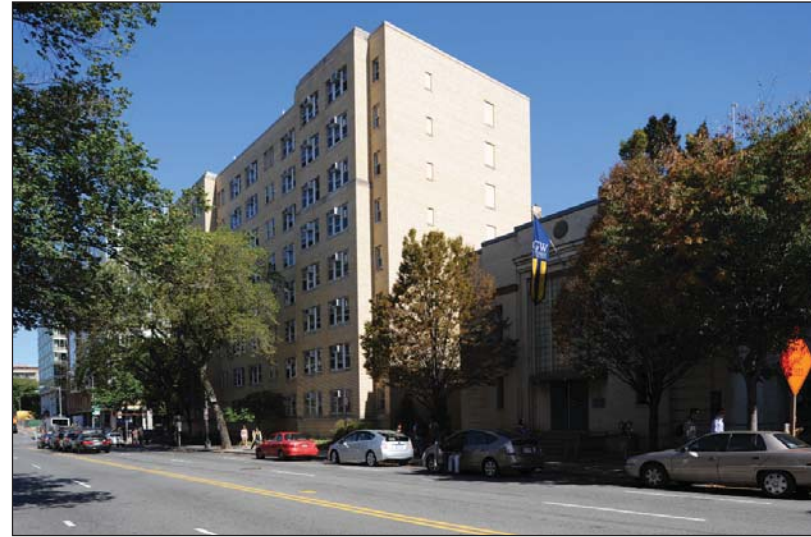
2.) 23 rd Street looking North toward Building K (demo.) and JBKO in background
