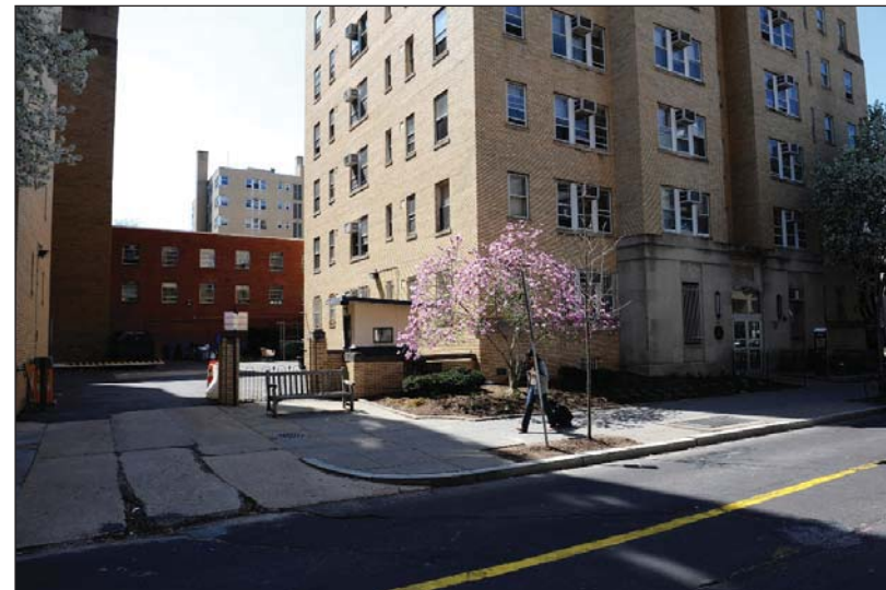
8.) Service Area behind JBKO Residence Hall (right) with Building K and parking garage behind (mid-ground, demo.)
