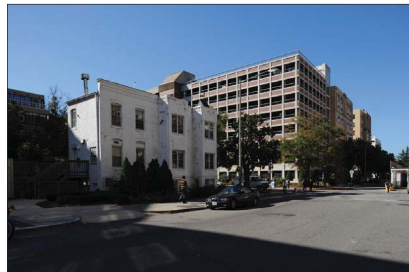
8.) Corner of Eye and 22 nd Streets looking toward Square 55 (right), across the site of future development (left).
