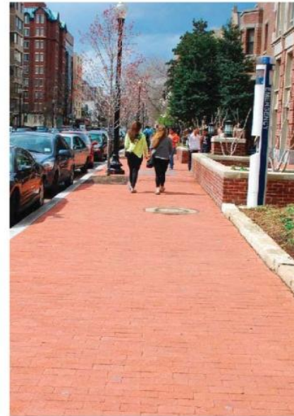
BRICK WALK (Located on H Street and Eye Street)
