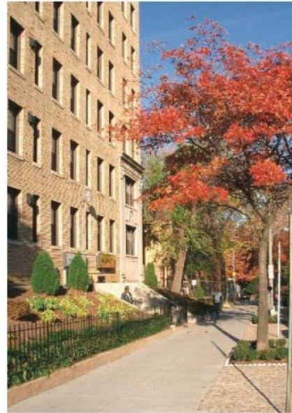
CONCRETE WALK (Located on 22nd Street and 23rd Street)
