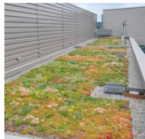
Green Roof & Cistern
