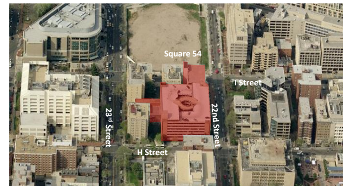
Aerial View Looking North
