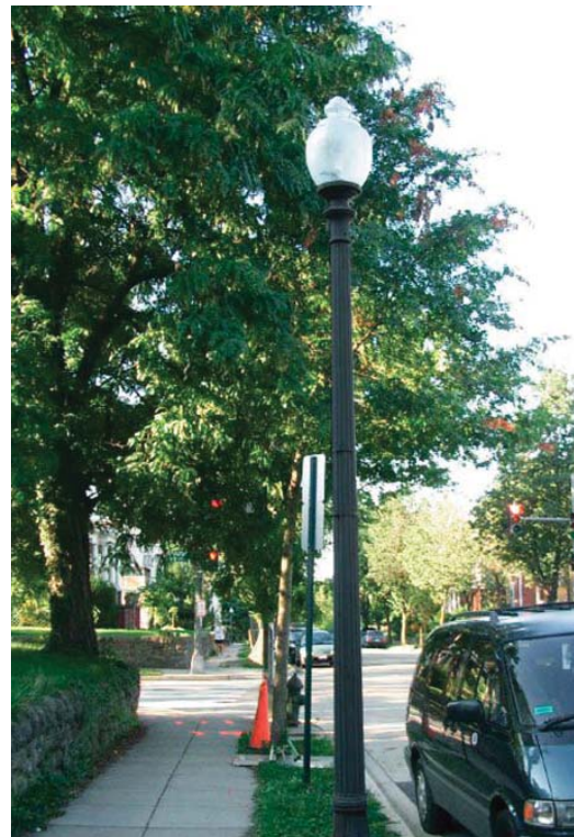
WASHINGTON GLOBE STREETLIGHT
