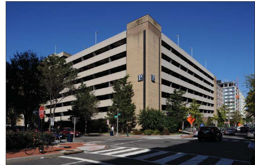
6.) Corner of 22 nd and H Streets looking Northwest toward the Parking Garage (demo.)
