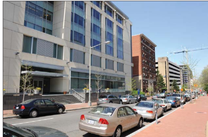
4.) 22 nd Street looking North through GW Campus toward Square 55 (right-of-center, distant)
