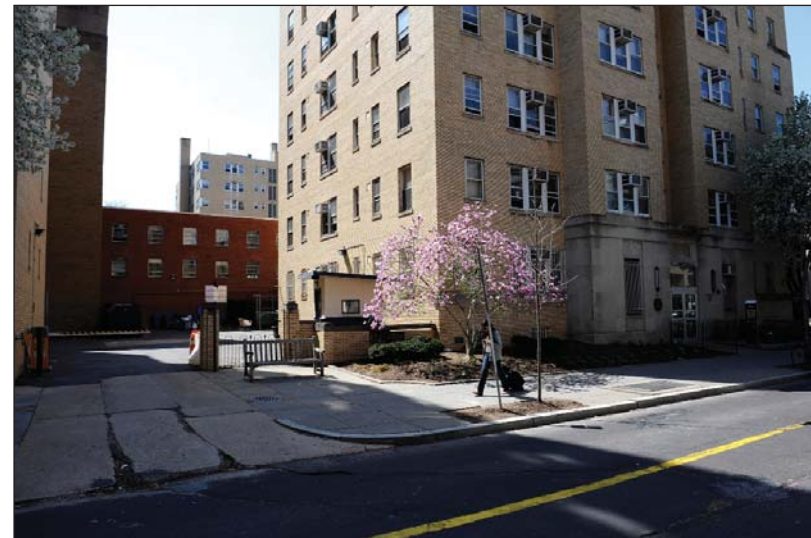
8.) Service Area behind JBKO Residence Hall (right) with Building K and parking garage behind (mid-ground, demo.)
