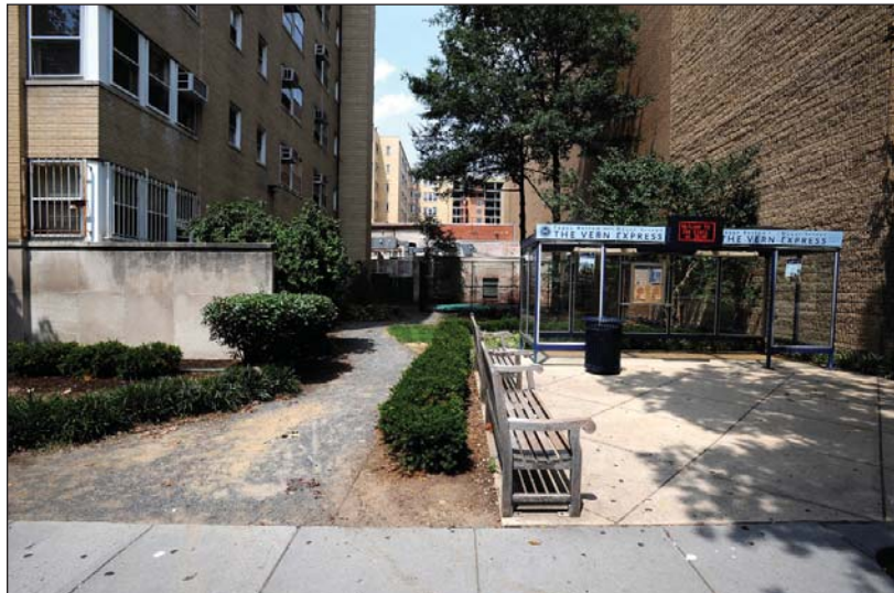
4.) H Street court between Fulbright Residence Hall (left) and Parking Garage (right, demo.) with current shuttle stop
