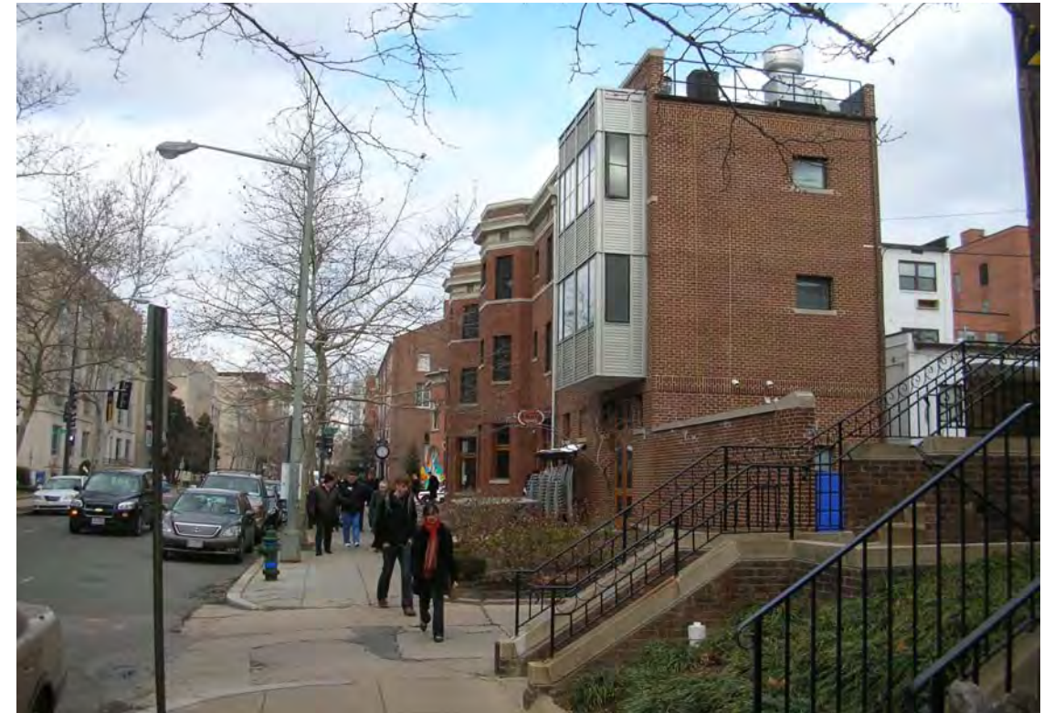
VIEW OF 21ST STREET SIDEWALK LOOKING NORTH
