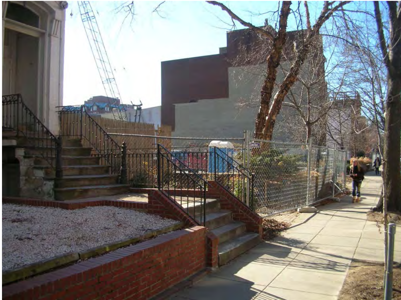
VIEW OF G STREET SIDEWALK LOOKING WEST
