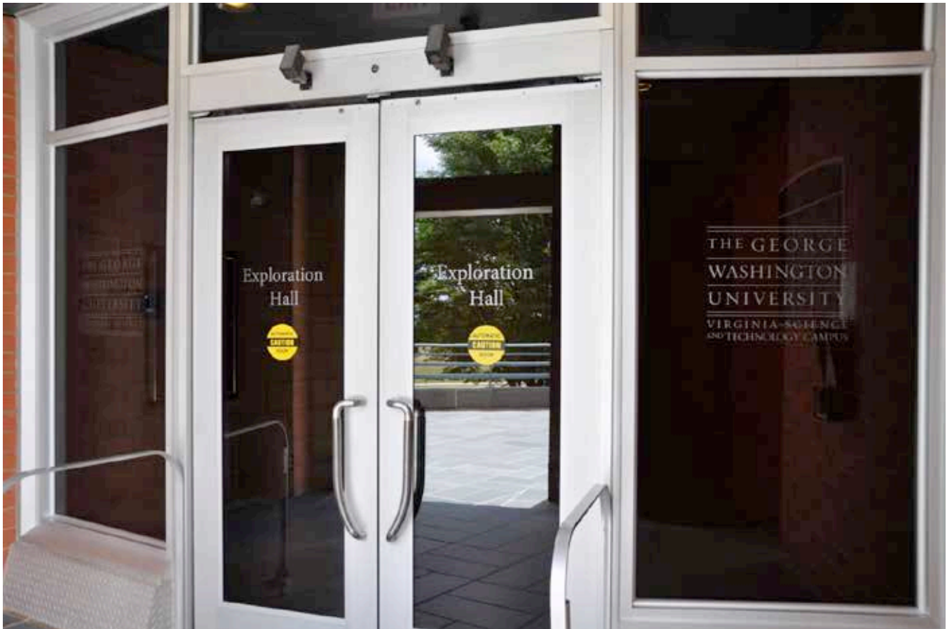
Existing Glass-Mounted Signs at Exploration Hall
