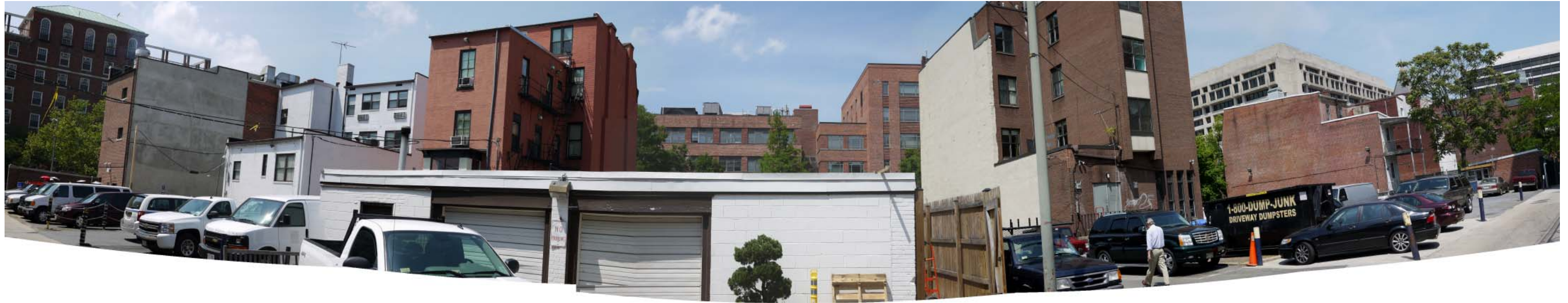
5. VIEW OF SITE FROM ALLEY, MID-BLOCK, LOOKING NORTH
