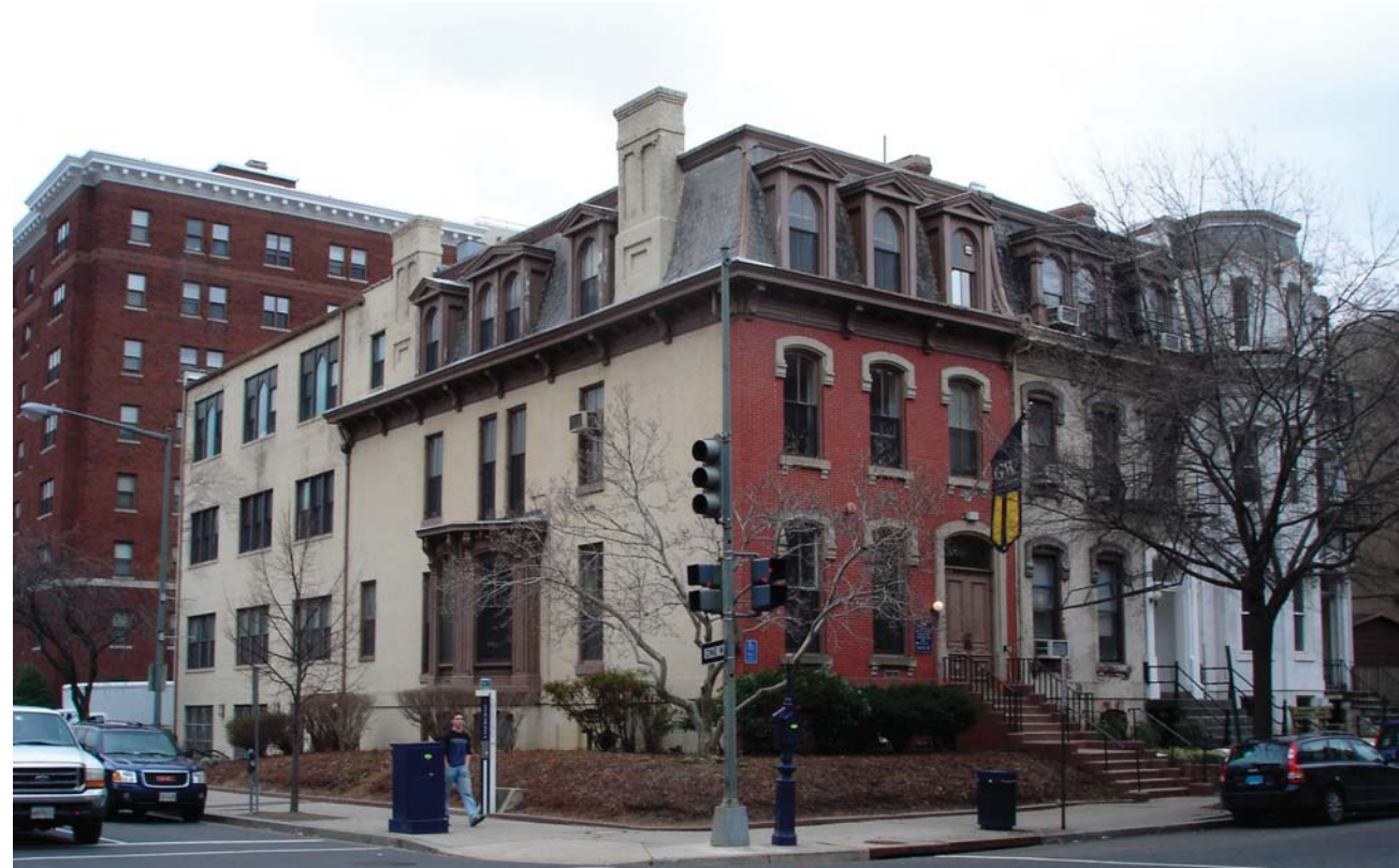
2. VIEW OF ADJACENT ROW STRUCTURES AT G AND 20TH STREETS LOOKING SW
