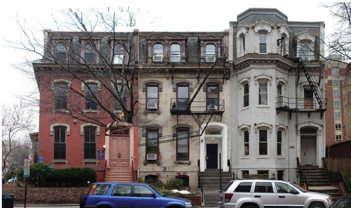
3. VIEW OF ADJACENT ROW STRUCTURES FROM G STREET
