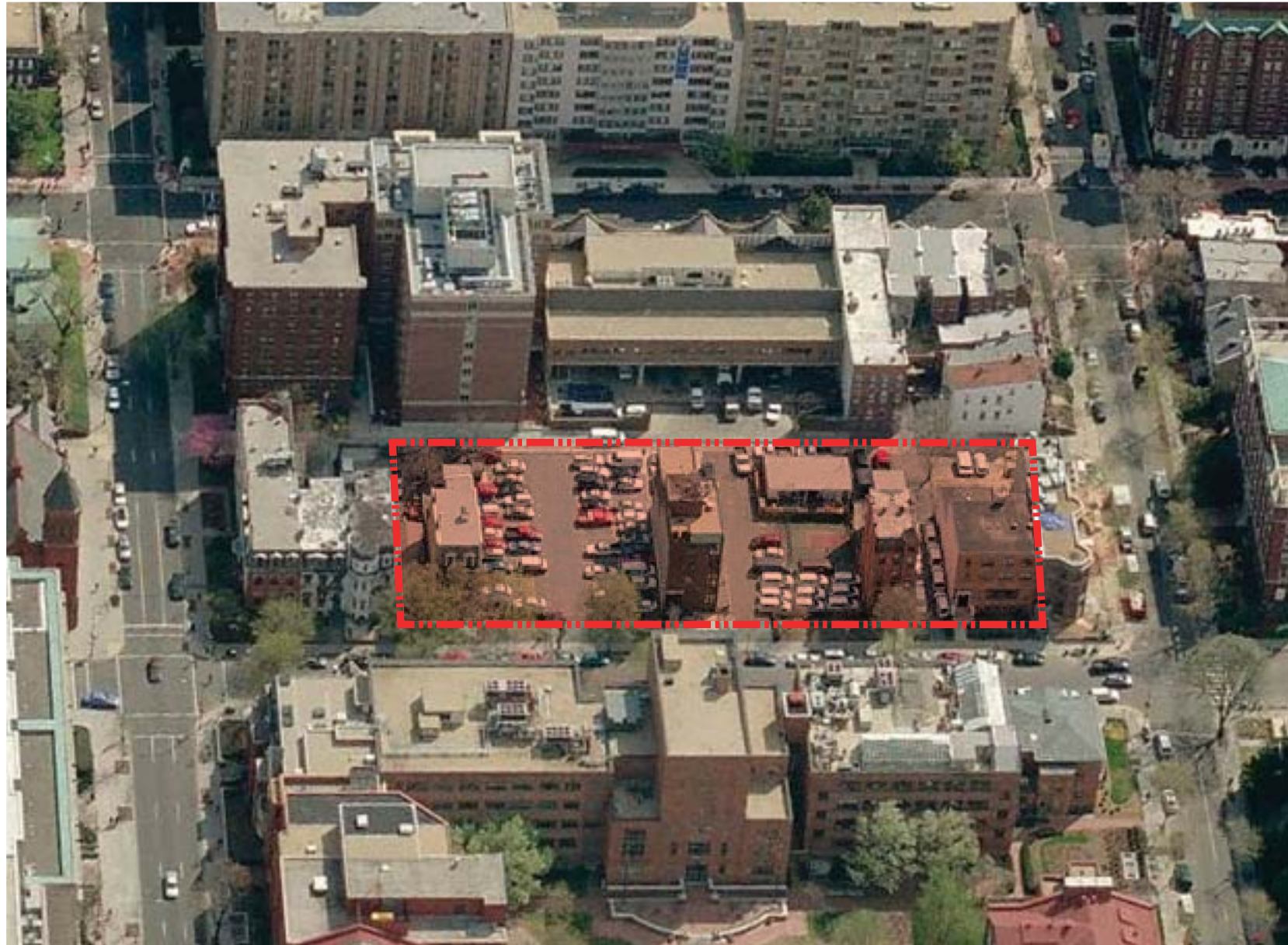
AERIAL VIEW LOOKING SOUTH
