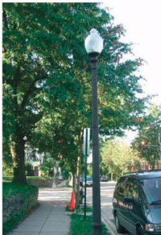
WASHINGTON GLOBE STREETLIGHT
