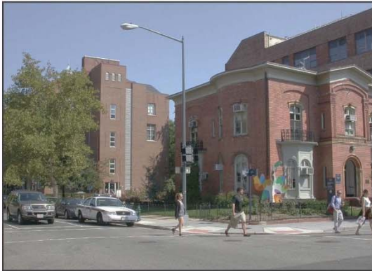
1. VIEW OF SITE, LOOKING NORTHEAST
