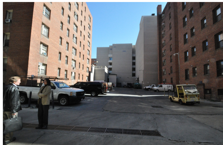
15.) View from service area, looking east towards Marvin Center loading dock. Rear of Schenley and Crawford Halls to the right. The West End rear to the left.
