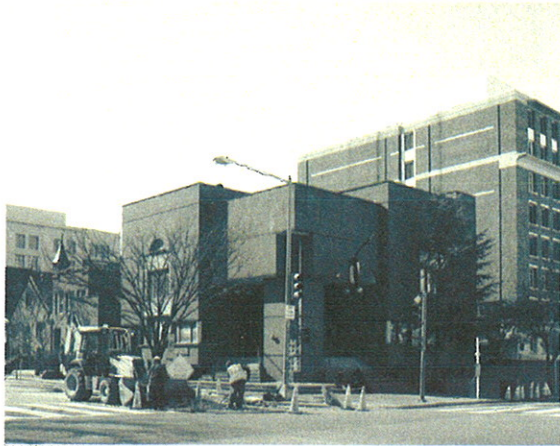
EXISTING HILLEL BUILDING
