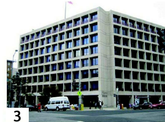
3 2100 PENNSYLVANIA AVE EAST
