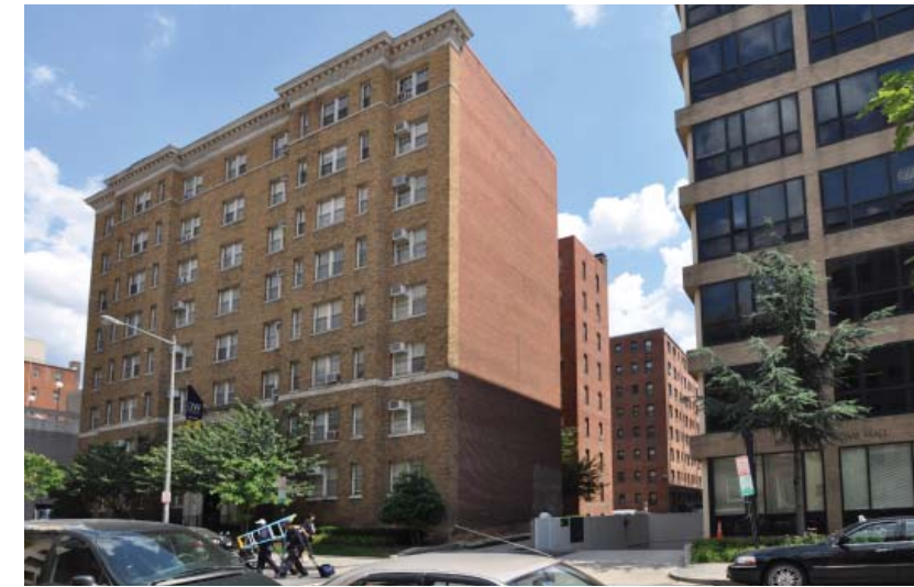
11.) View from across Eye Street, looking southeast at the service alley between The West End and Academic Center.
