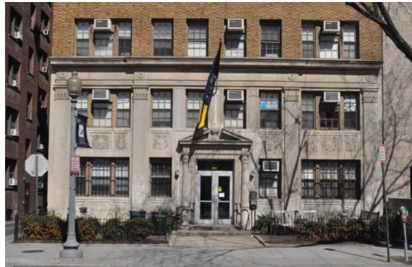
5.) View of Crawford Hall entry looking north from across H Street.
