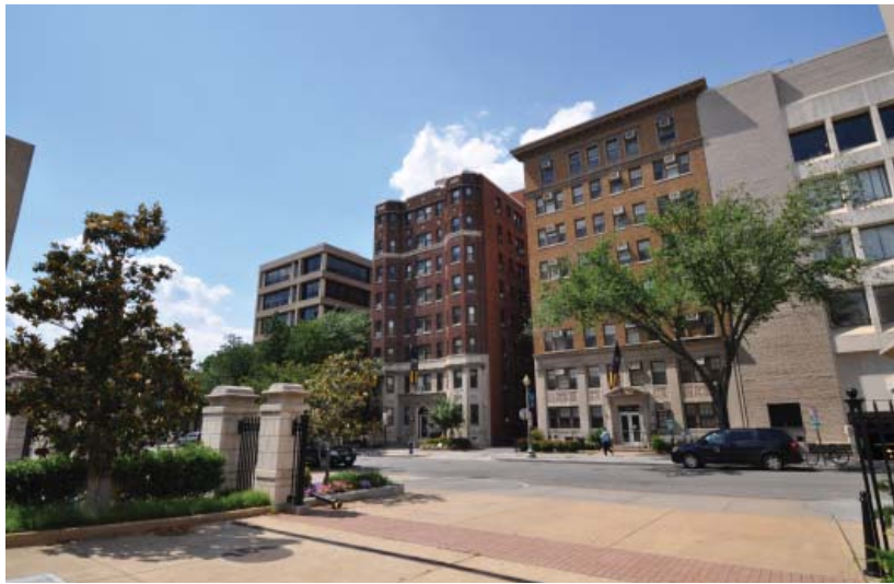
1.) View across H Street, from Kogan Plaza, looking north at Schenley and Crawford Halls.
