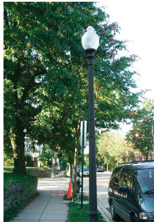
WASHINGTON GLOBE STREETLIGHT
