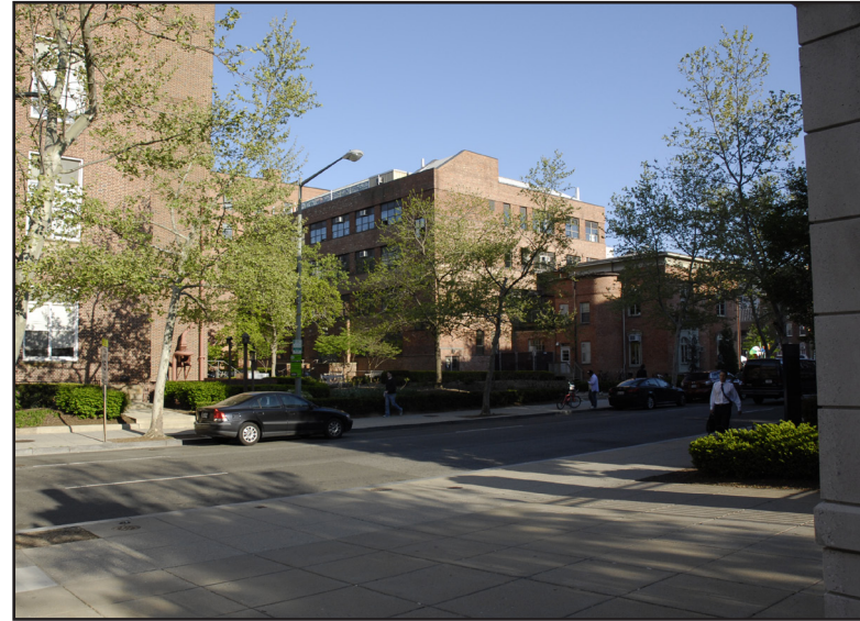
3. VIEW OF SITE, LOOKING SOUTHEAST
