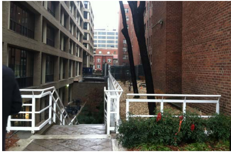
Existing alley condition
