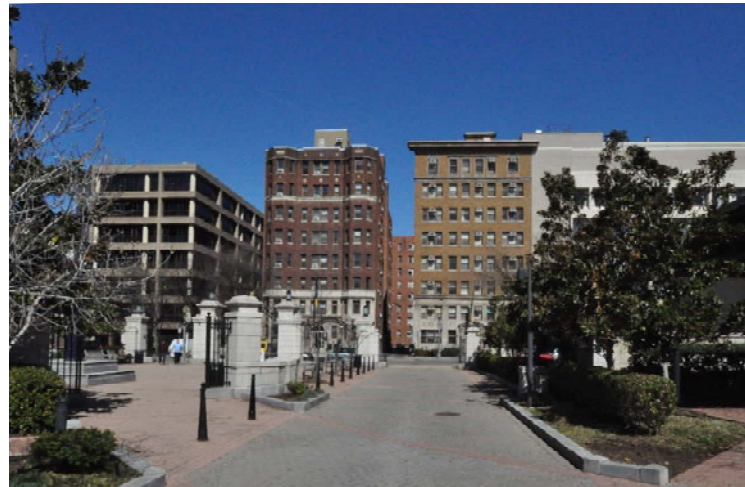
2.) View from Kogan Plaza, looking north at Schenley and Crawford Halls.
