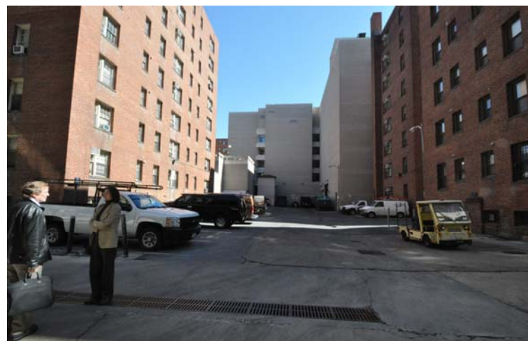
15.) View from service area, looking east towards Marvin Center loading dock. Rear of Schenley and Crawford Halls to the right. The West End rear to the left.
